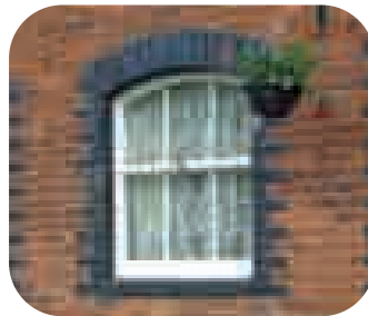
5. Victorian Blue Brick Window detailing and Lintel
