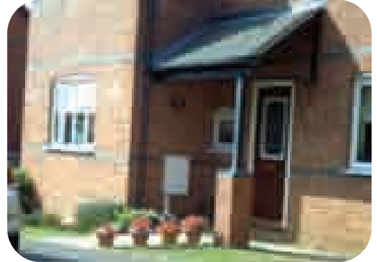
Example of rebated traditional windows
