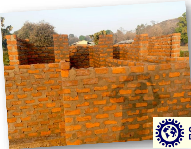
Building latrines on site
